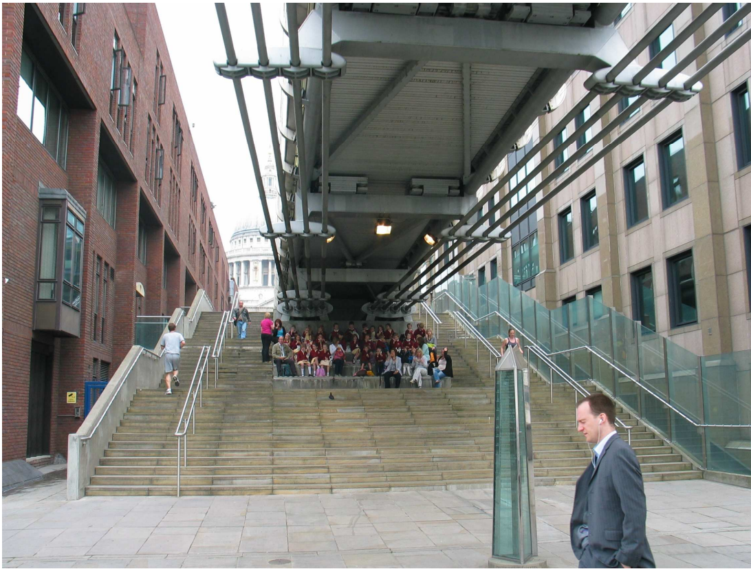
Space under the Millennium Bridge
